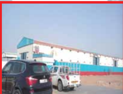
DANA STEEL - UAQ Branch
