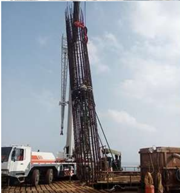
Super-Cell Technology, Sudan Port of Africa 1200mm ring-type for 8MN load and 1500mm combined for 10MN load, year 2015
