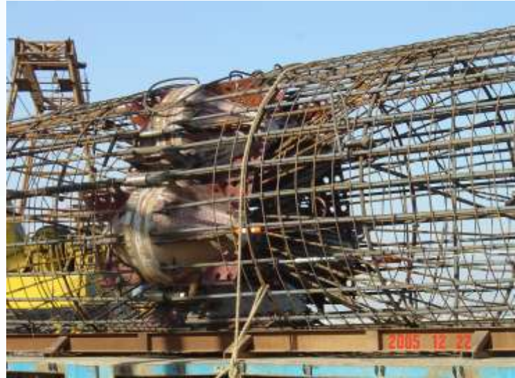
Hangzhou Bay Bridge (Longest Cross-Sea Bridge ever built, 70 MN load, year 2006)
