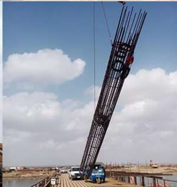
Super-Cell Technology, Sudan Port of Africa 1200mm ring-type for 8MN load and 1500mm combined for 10MN load, year 2015
