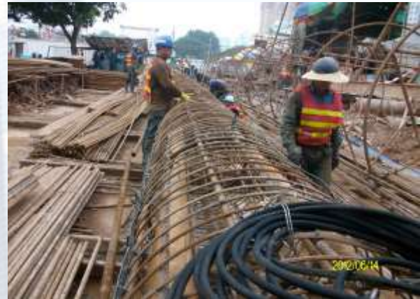
Qingzhoufang Residential Building, Macau, China (1,000 mm dia pile, 11.7 MN load, year 2012)
