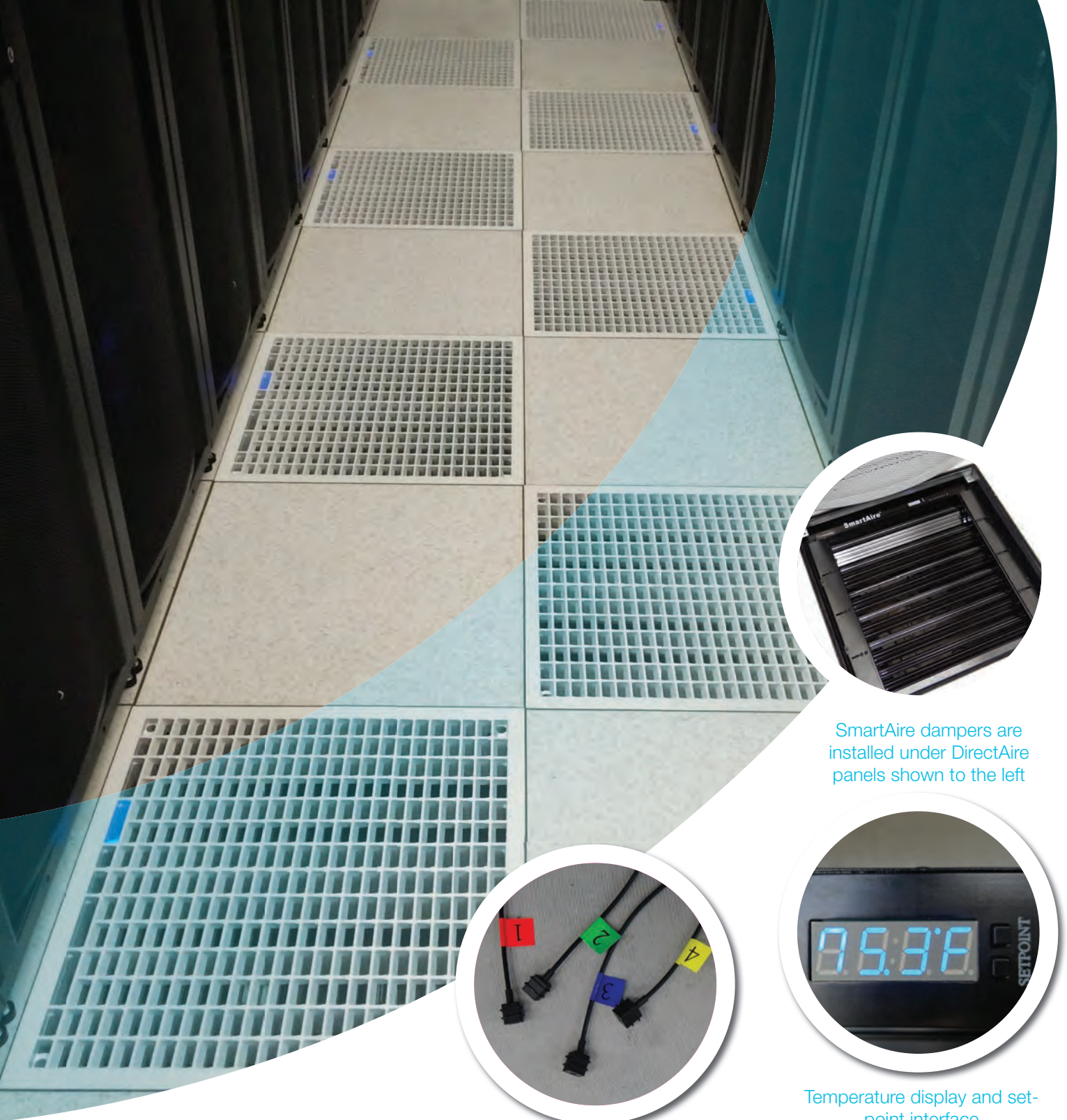
Four temperature sensors are mounted to the face of the rack
