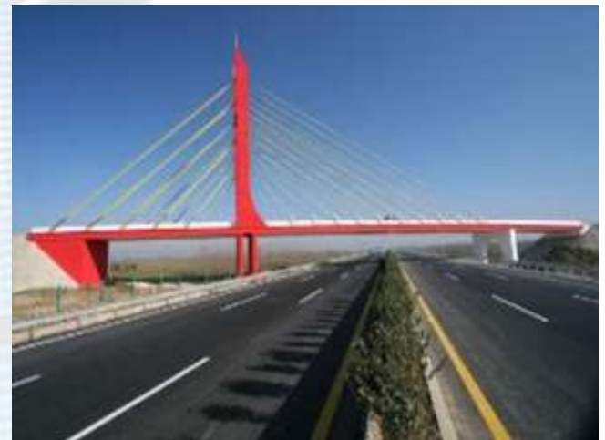
Nandeng highway of China Railway 5th Bureau Group
