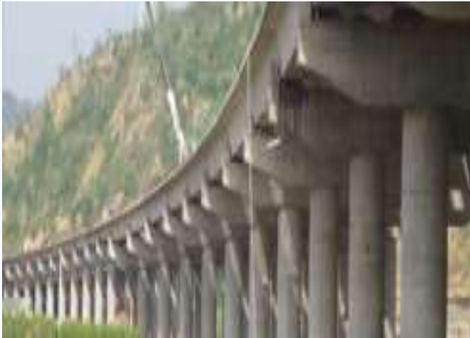
Shitian highway No.31 Subproject of Eastern Alliance Construction Engineering Co.
