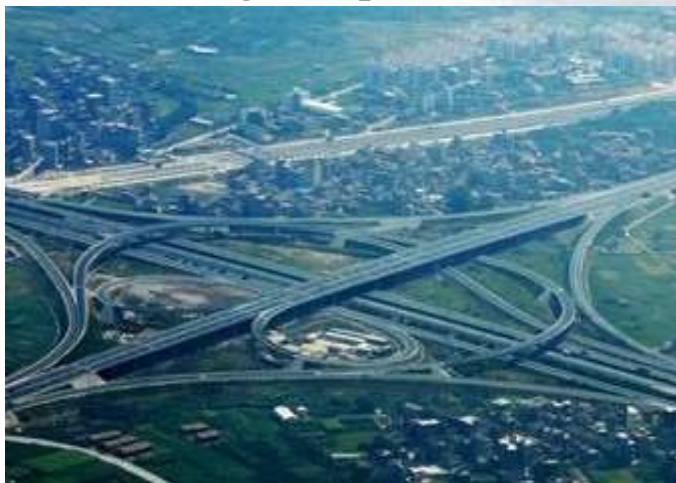
Puxiu highway of China Road and Bridge Corporation
